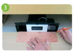
Remove the front panel from the Sweepovac unit. Place the template on the kickboard in the centered location as shown. Draw a line around the 3 sides.
