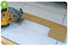
Use the jigsaw to accurately cut along the center of the line
